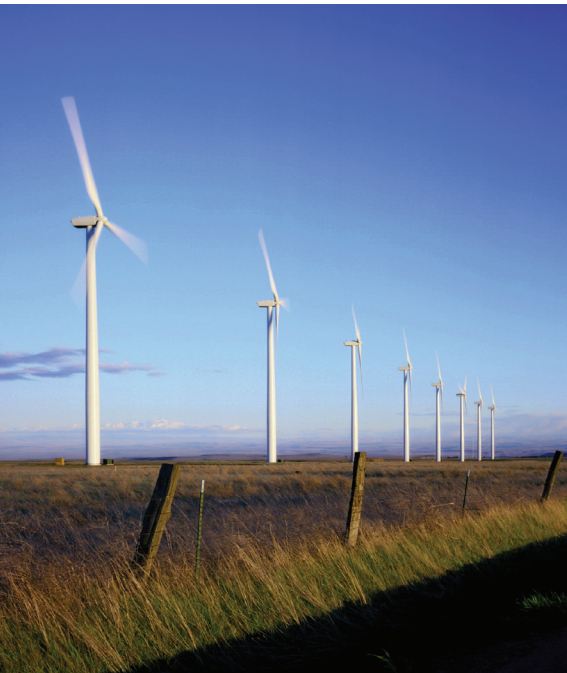
PPM ENERGY (BIG HORN WIND POWER PROJECT NEAR BICKELTON, WASHINGTON)
